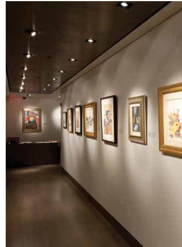
The corridors are also used as exhibit space, but low ceiling height prevented the use of track lighting. Recessed MR16 downlights are used here in the entry hall.
