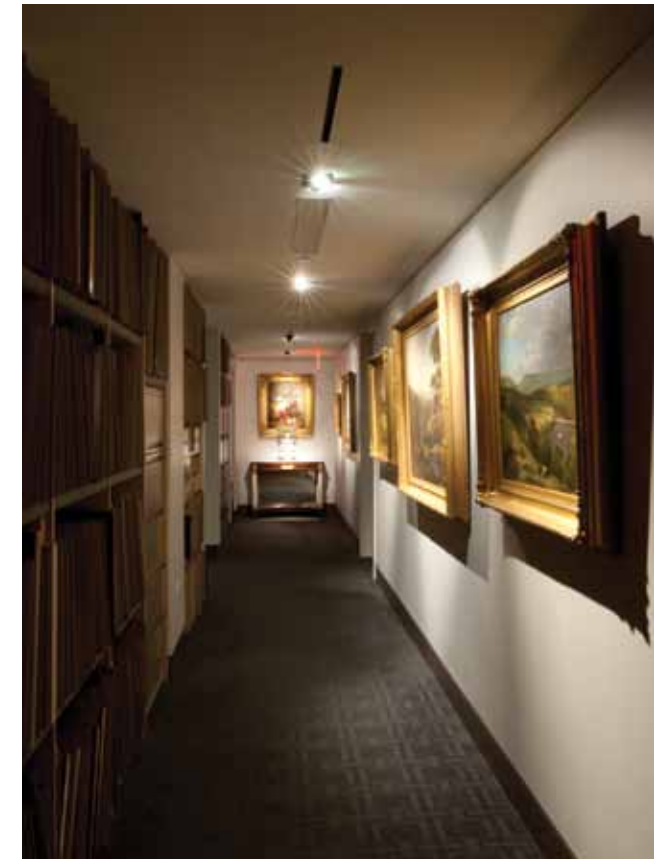
As is the case in the galleries, the linear air diffusers align with the MR16 and fluorescent lighting for a crisp, unified appearance along the ceiling plane.
